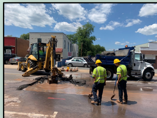
Main Street Water Main Break & Repair
