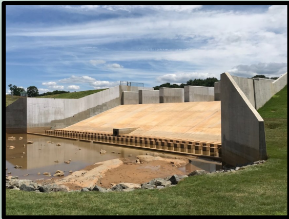
Mountain Run Lake Dam Rehabilitation Construction 2019
