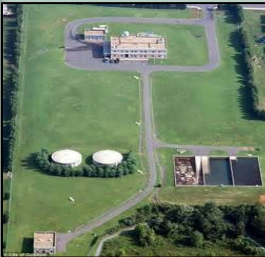
Water Treatment Plant
