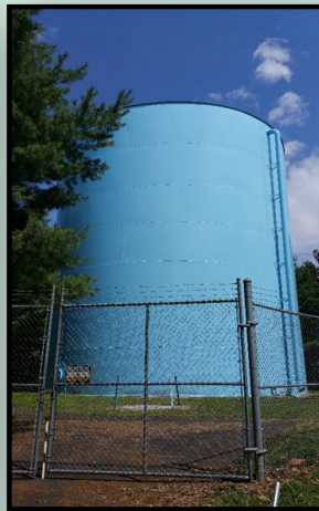
West Ground Storage Tank
