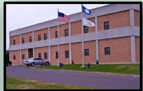
Water Treatment Plant 816 Woodview Road
