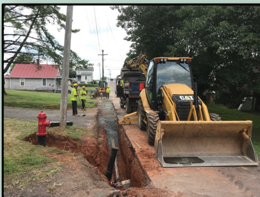
Bickers Street Water Line Replacement
