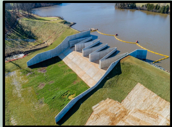
Lake Culpeper Dam Rehabilitation Construction 2019
