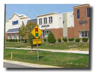
An example of facade articulation used to break up the mass of a bigbox store. This example is a side facade facing a residential area.
