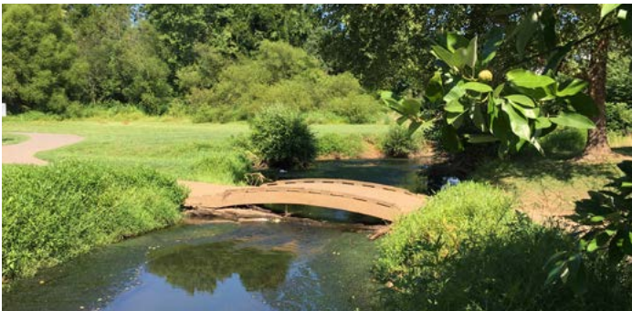
Existing low water bridge
