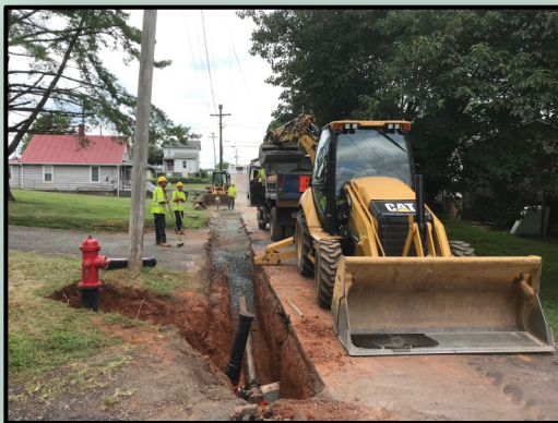
Bickers Street Water Line Replacement
