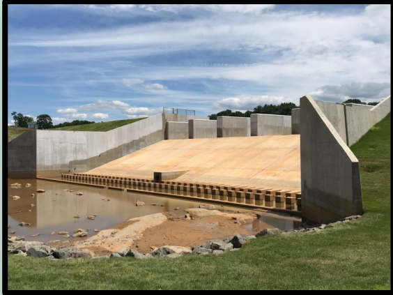
Mountain Run Lake Dam Rehabilitation Construction 2019
