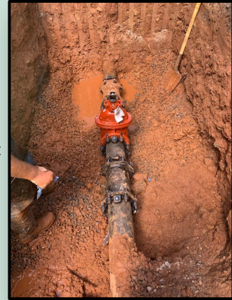
Oaklawn Drive Valve Replacement
