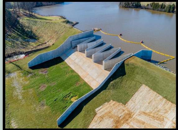
Lake Culpeper Dam Rehabilitation Construction 2019
