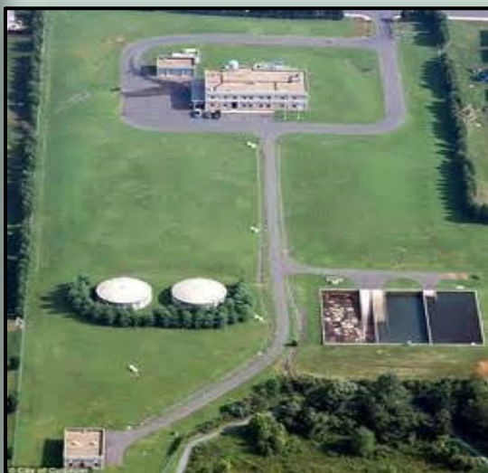
Water Treatment Plant
