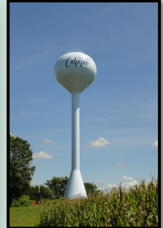
Pedisphere Storage Tank
