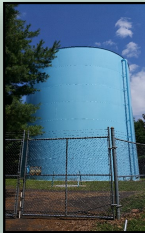
West Ground Storage Tank
