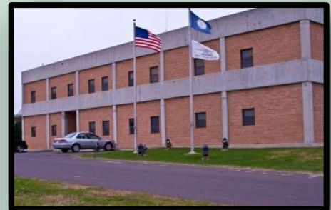
Water Treatment Plant 816 Woodview Road
